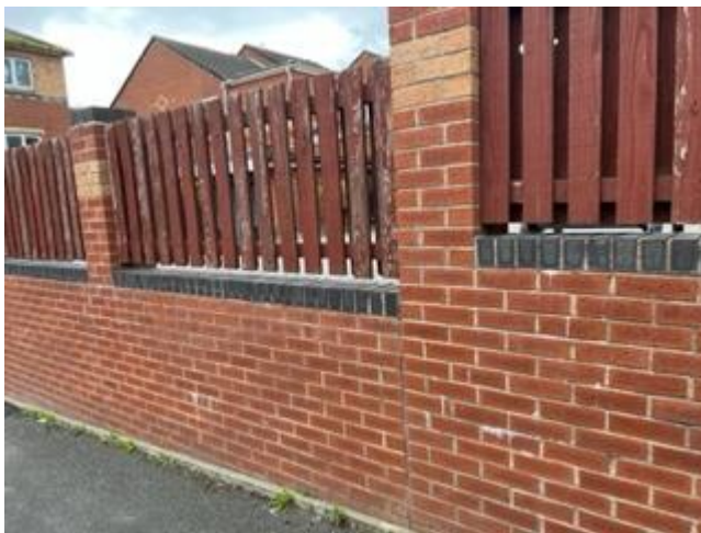
Back garden of a neighbour along the same path further up
